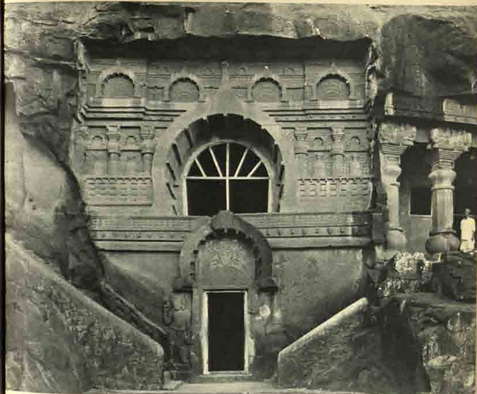
108. Façade of the chaitya-griha at Nasik (pp. 48 and 169)
