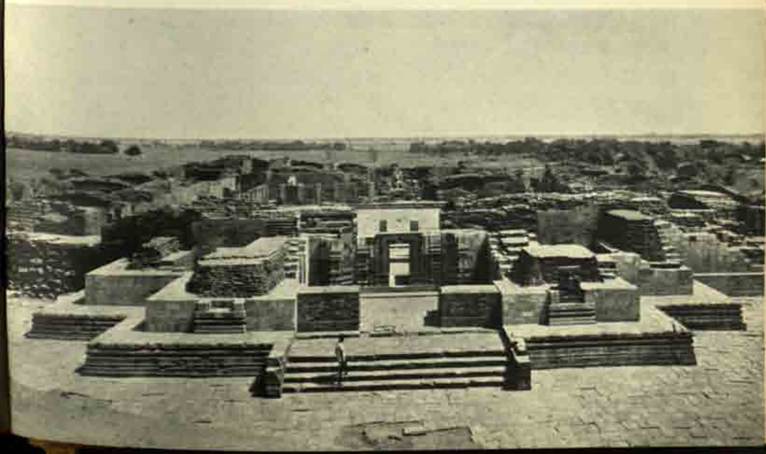
138. Monastery I at Ratnagiri (pp. 228-30)
